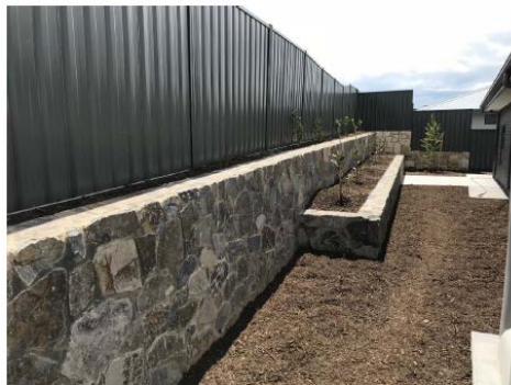
Image 6. Rear retaining wall solution with fencing above.
