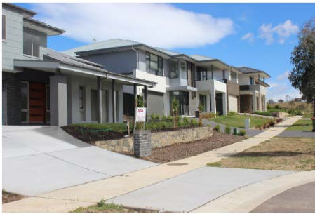
Image 1. A typical streetscape which shows a combination of front retaining walls used or a battered front lawn to take up the lot grade.
