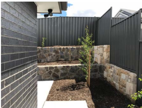
Image 5. Rear stepped retaining walls with side and rear fencing to a steep lot.
